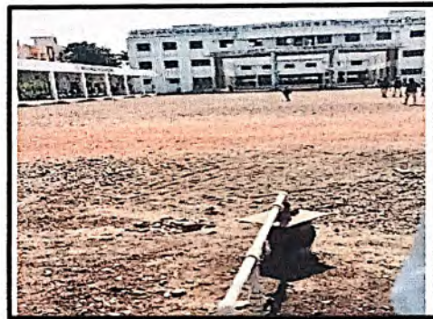
Bore well Charging
