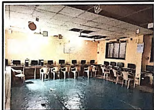
Lighting System at campus
